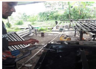
Figure 17: Measuring and Arranging Hollow Bar for Spring Basement
