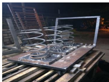
Figure 18: Welding Spring Basement
